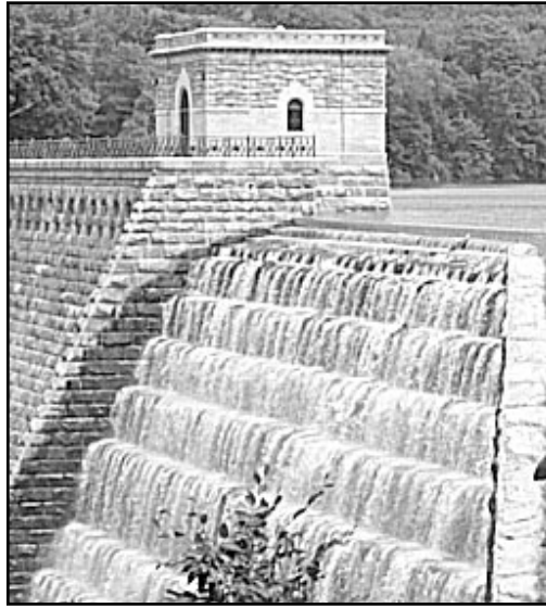
Spillover from the Amawalk Reservoir
